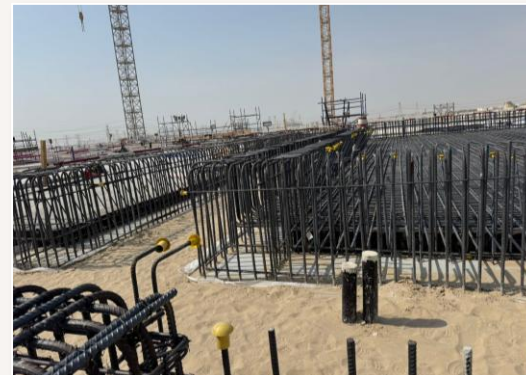
Rebar & Concrete Works
